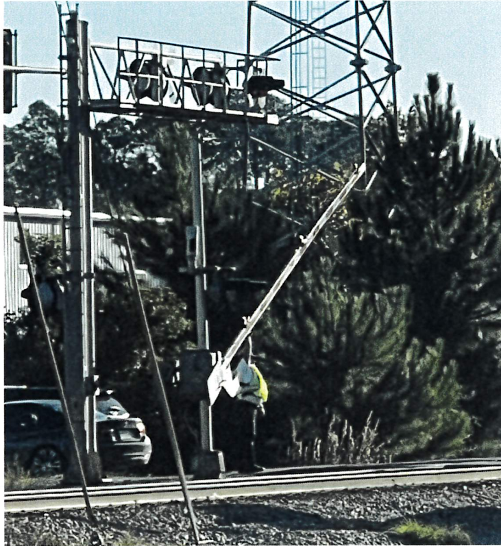
Image 3: OSPD Officer holding up the CSX Railroad Crossing gates with his hands to allow multiple cars to pass under; photo taken on Wednesday, November 12, 2025 at 7:51am.
