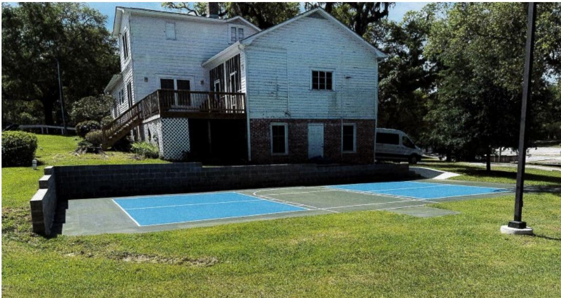
Figure 3. Existing Sport Court
